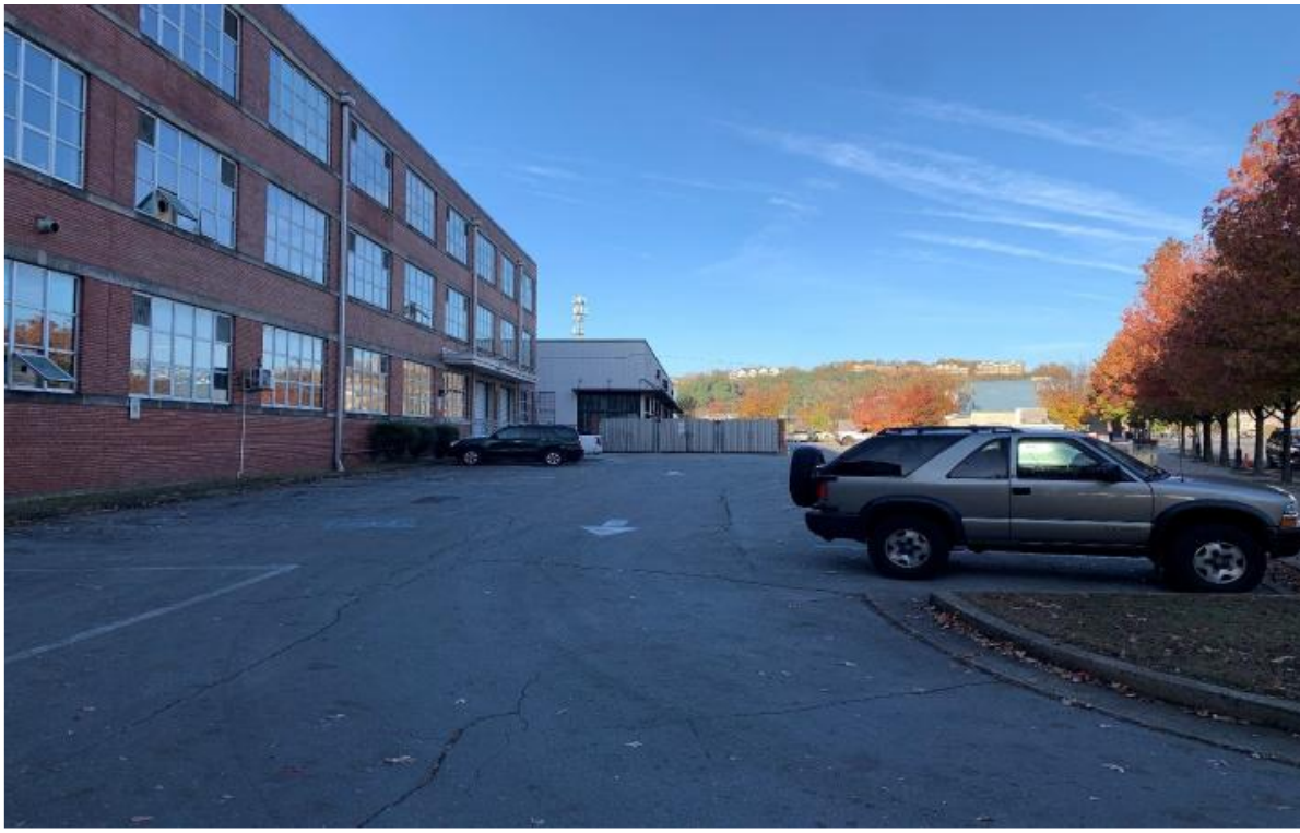
PARKING / LOADING AREA
